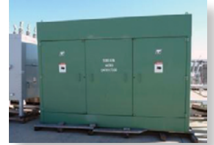
Pad-mounted transformer
