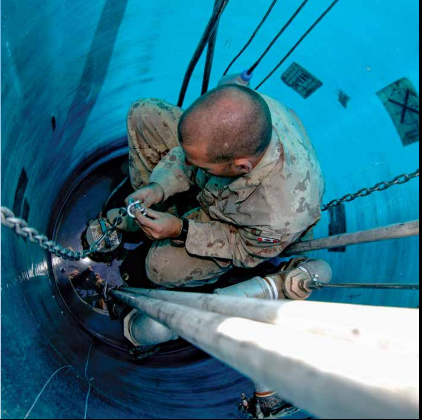
Master Corporal Trevor Dalheim, a Water Fuel and Environment technician with Task Force Afghanistan at the Provincial Reconstruction Site, attaches a chain to a lift station pump in November 2005.
