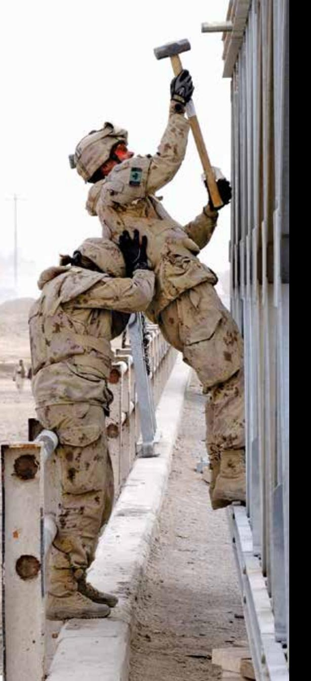
Engineers work on assembling a Mabey-Johnson bridge (a portable pre-fabricated truss bridge) in Kandahar, in March 2010.
