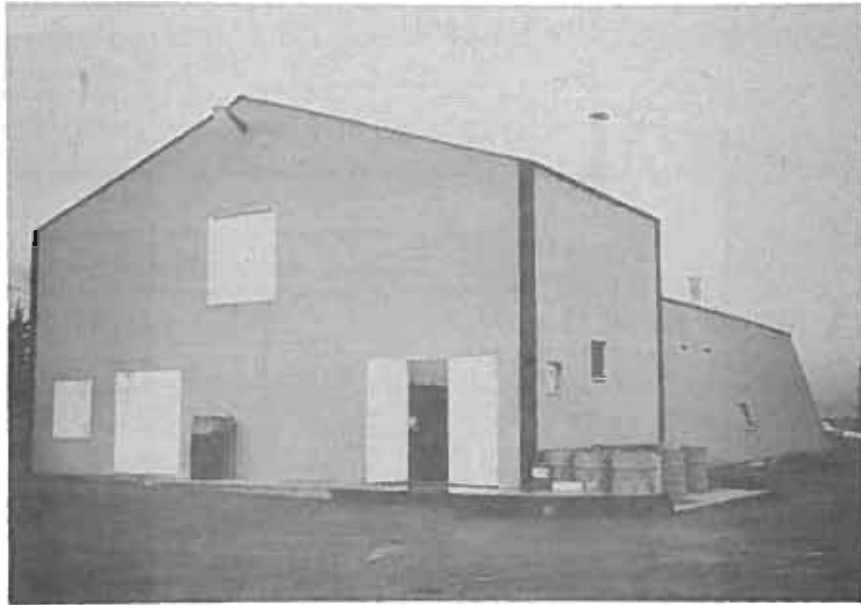
Fig. 3: Upgraded Facility - Exterior View.
