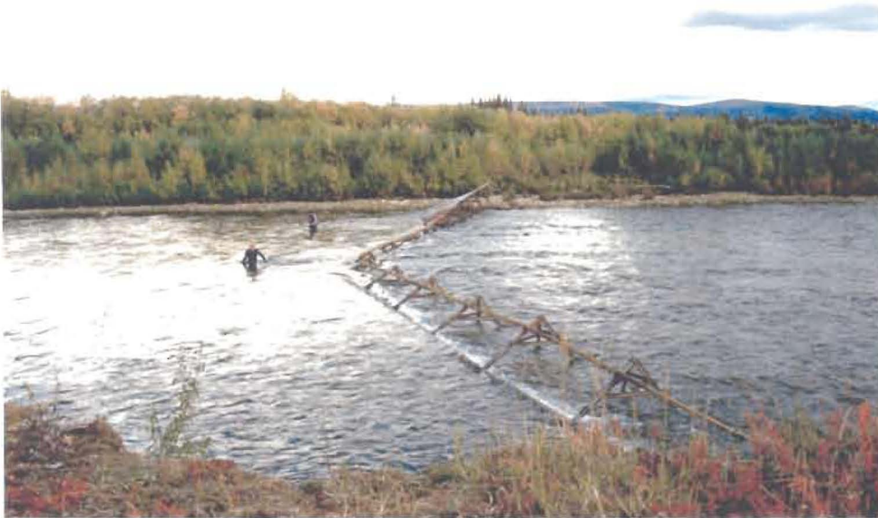
Photograph 1. Typical construction of the Fishing Branch River weir.
