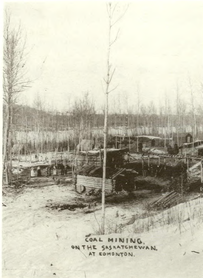
139. Coal miners' accommodation, Alberta.
