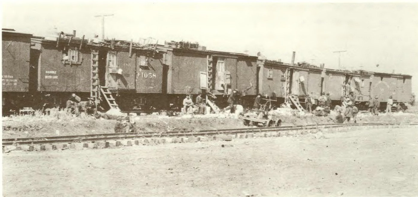
127. Bunk cars for railway construction workers.
