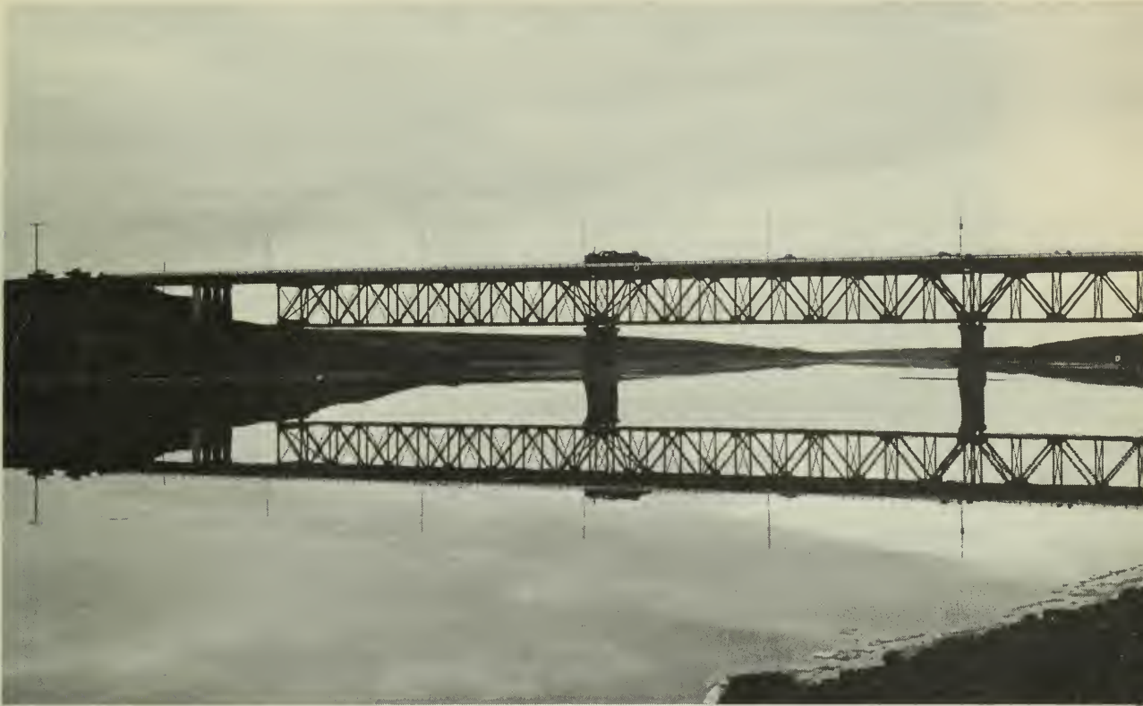
Construction bridge at South Saskatchewan River damsite gives access to structural area.
