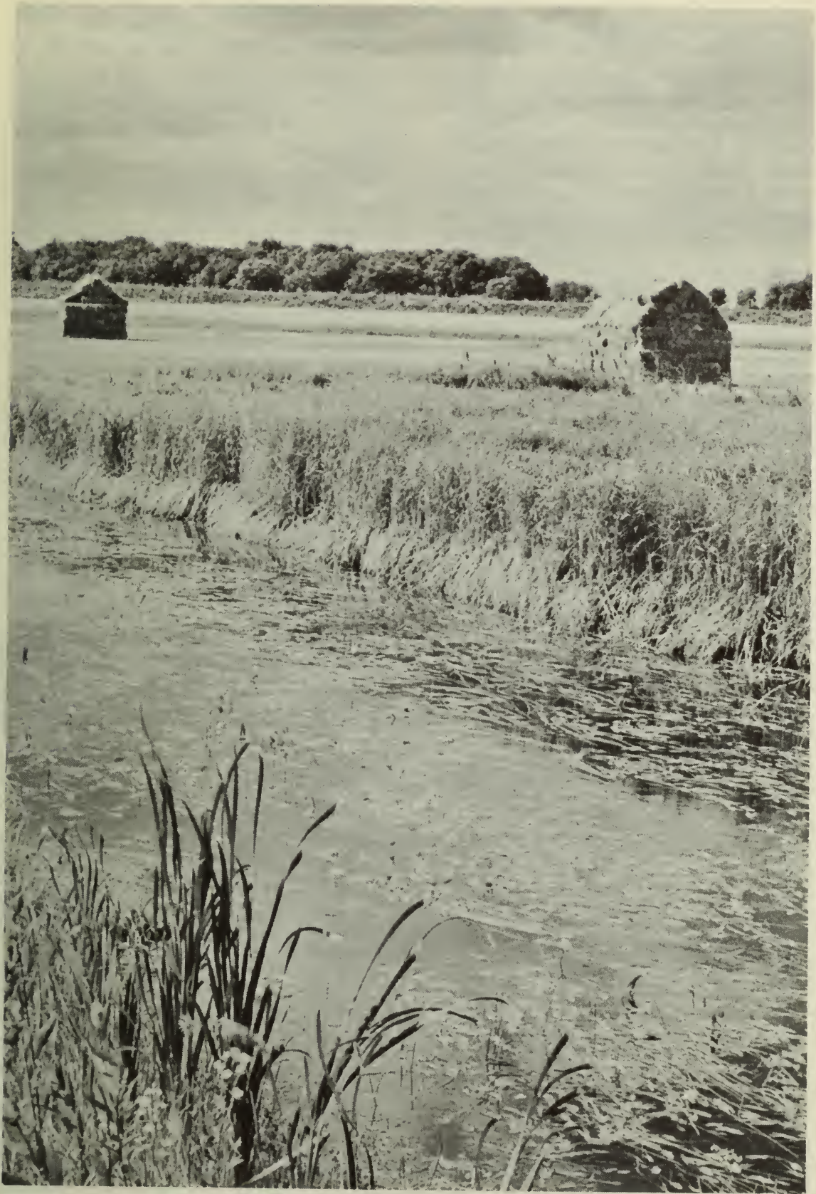
Pasquia River diversion channel in Manitoba is part of the Saskatchewan River Reclamation Project.
