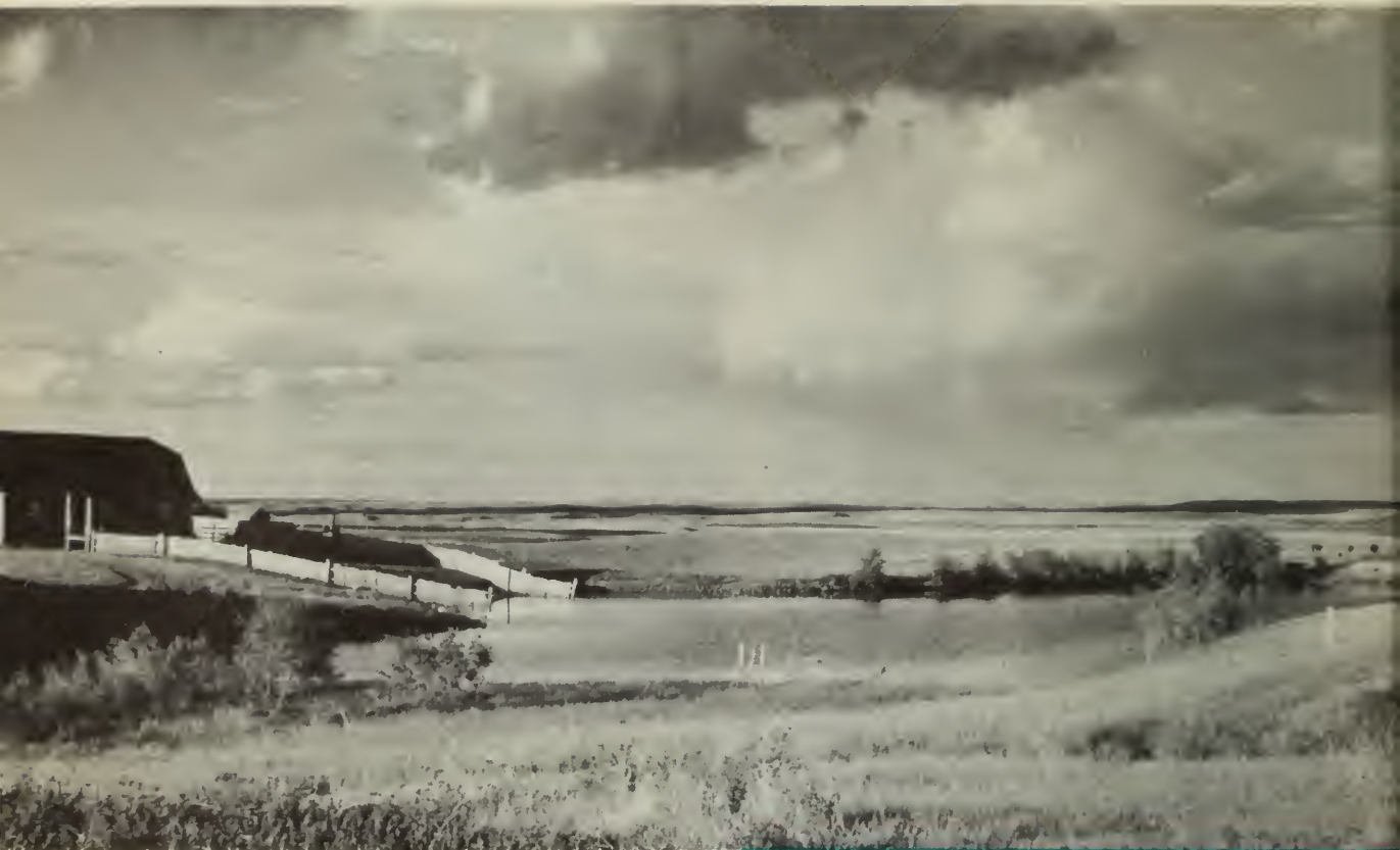
Typical individual farm-sized stockwatering dam built with PFRA assistance.
