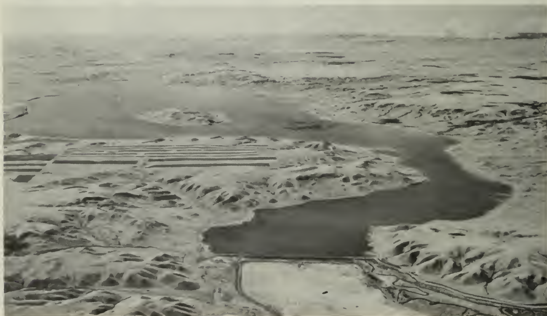
East Dam, Cypress Lake Reservoir, Saskatchewan. Reservoir is largest of 11 PFRA projects utilizing water from Cypress Hills.
