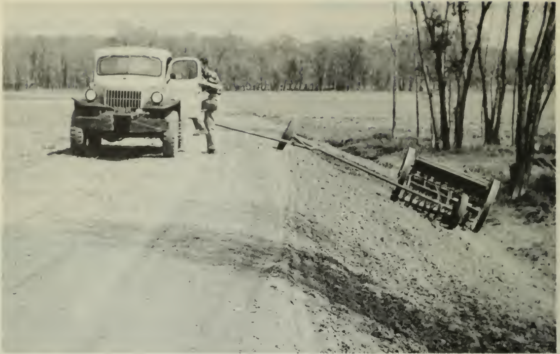
Dykes built by PFRA along the Assiniboine River are seeded for protection from erosion.
