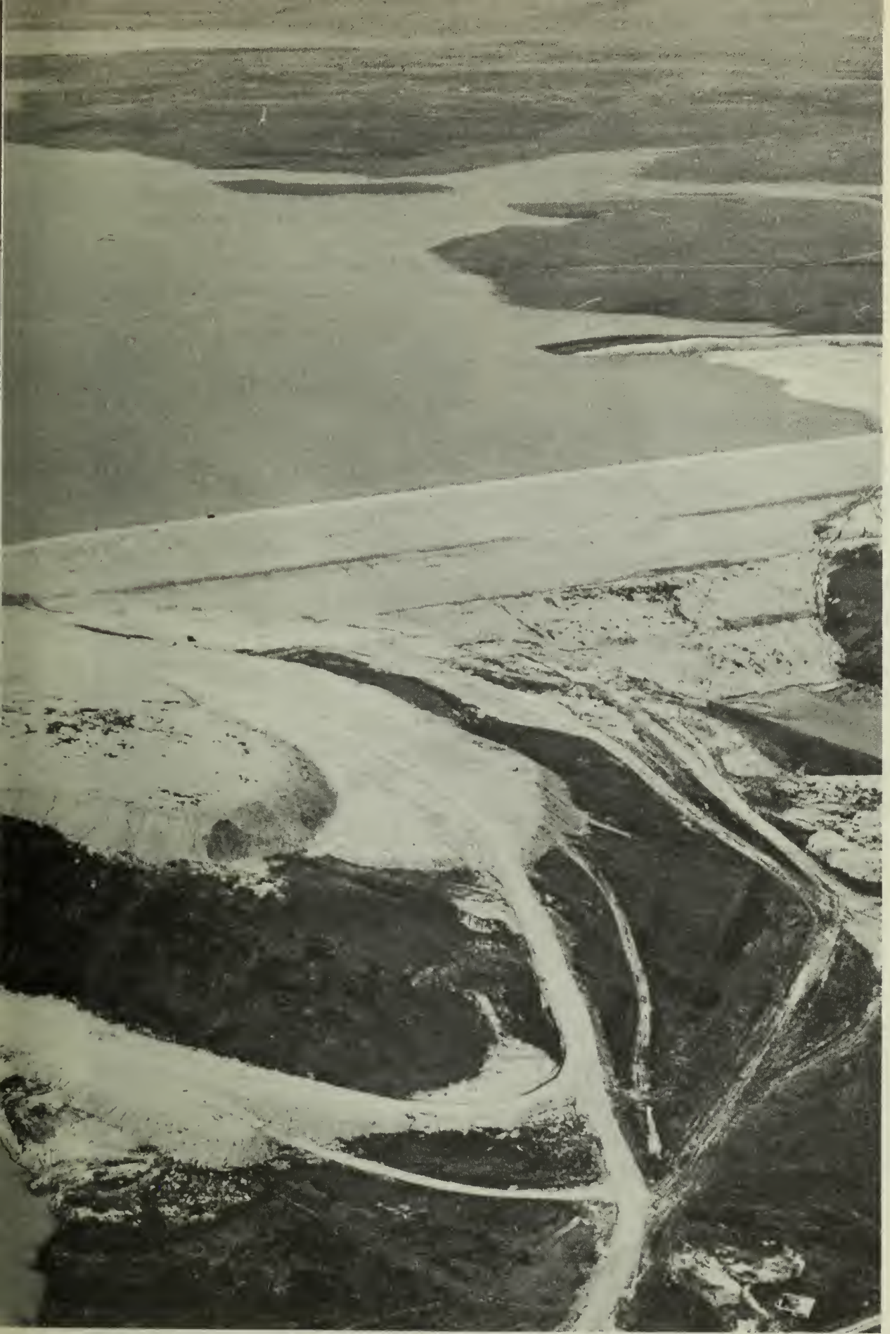
St. Mary Dam and Reservoir in southern Alberta.
