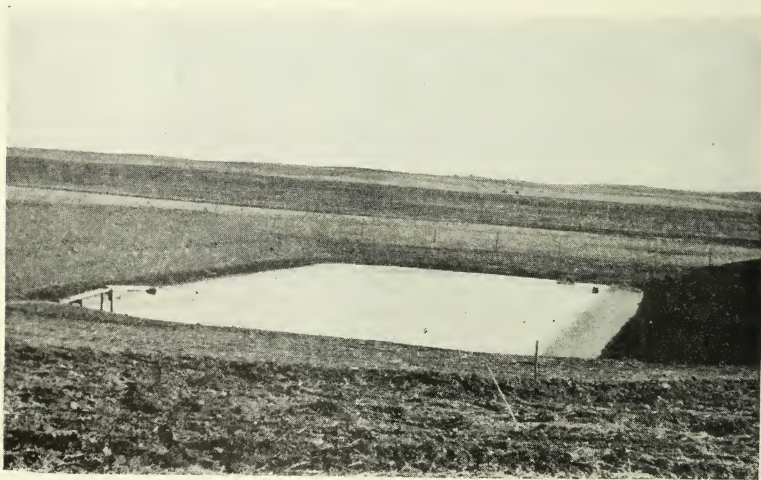
Typical farm dugout constructed under P.F.R.A.
