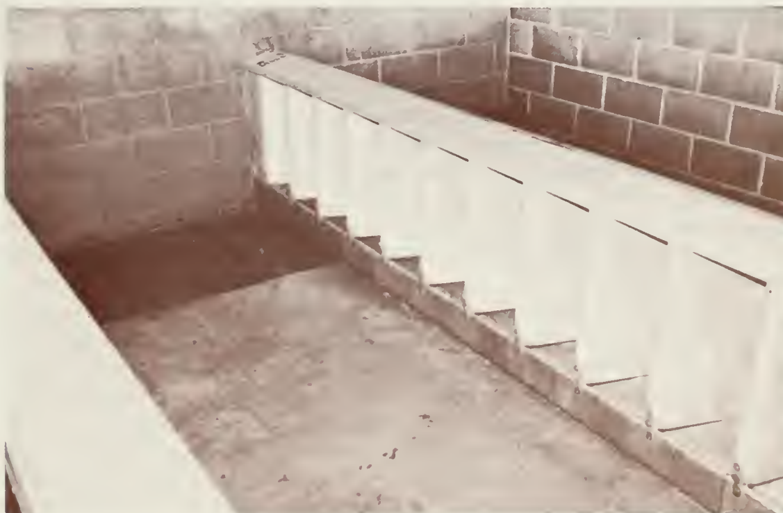
Figure 16. Strip feeder for a liquid feeding system.
