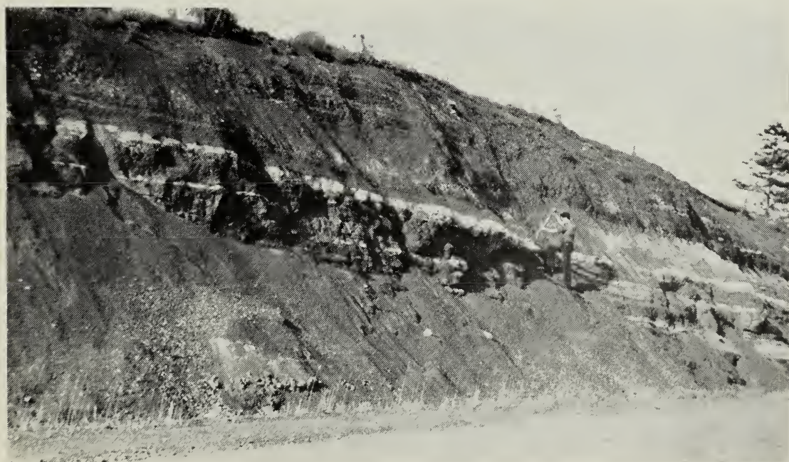
Fig. 4.—Road cut through the Lower Carboniferous formation near Kingsclear, N.B. The white streaks are light greenish coloured gypsum rocks, while the dark coloured material consists of bright red mud-stone, containing often as much as 80 per cent calcium carbonate.
