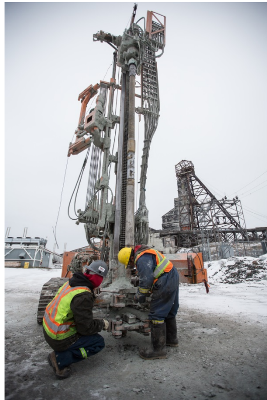
Geotechnical drilling
