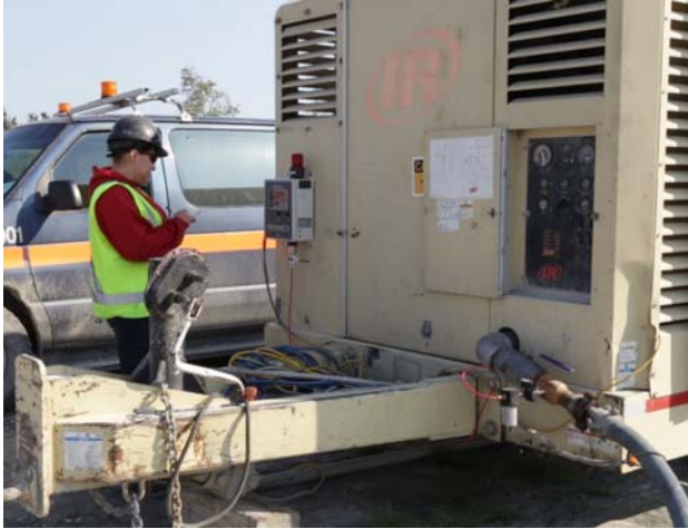
Checking a monitoring station on site.
