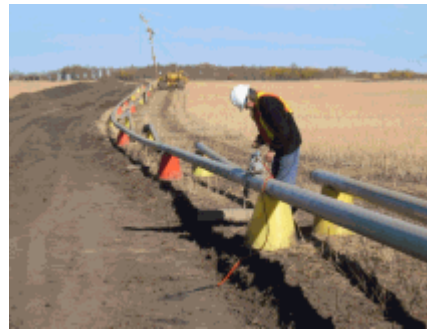
Image 6: NDT Pipeline inspection, using industrial radiography equipment
