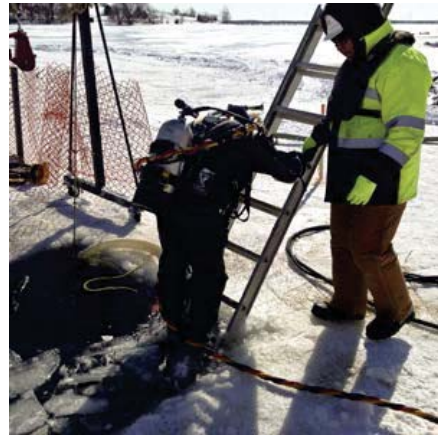
Between March 3 and 7, 2014, contract divers took the polar plunge to vacuum up approximately 16 m 3 of contaminated sediment from Navy Bay, using a 152-mm hose and pump.
