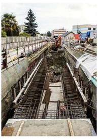
Utilities Corridor, CFB Esquimalt during construction. This underground concrete reinforced tunnel runs down the centre of the base's main road for over half a kilometre. The \$26-million corridor houses a wide range of utilities and permits easier maintenance and upgrades.
