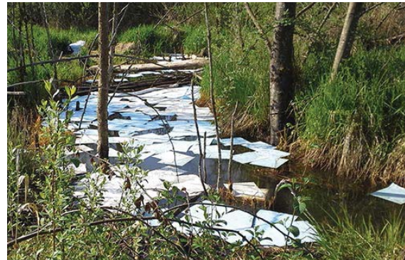
Spill pads are laid to contain the spread of fuel in the water
