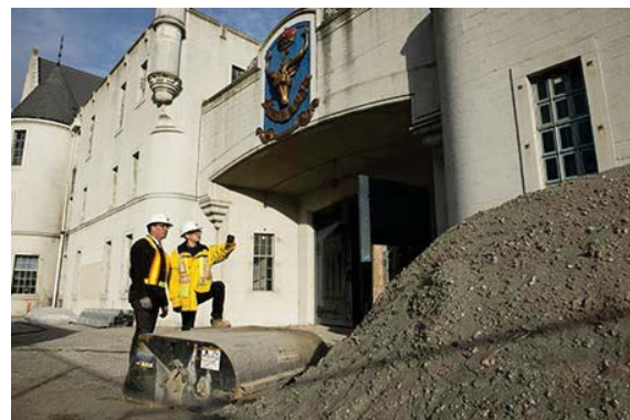
Steven Denault, Team Leader, Construction Services (left) with Julien Wong, Coordinator, Construction Services, two of the DCC staff who worked on the renovation and seismic upgrade of the Seaforth Armoury on the west side of Vancouver's busy Burrard Street Bridge.
