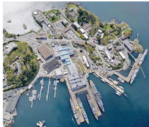
Aerial view of CFB Esquimalt, Canada's Pacific Coast naval base and home port to Maritime Forces Pacific and Joint Task Force Pacific Headquarters. The new A and B Jetty Recapitalization project will ensure the Canadian Armed Forces remain a first-class, modern military.
