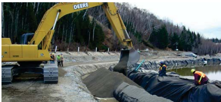
Installation of a passive recovery trench, or drain system, to cut-off and collect any free product (petroleum hydrocarbons) that may seep from the tank farm through the groundwater into the stillwaters.
