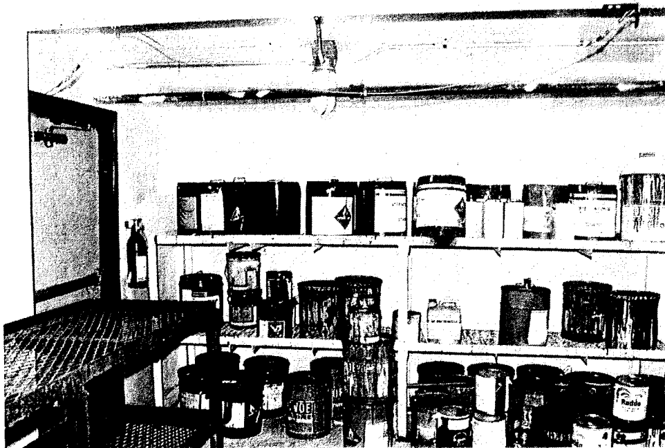
Sprinklered, fire resistant inside storage for paint and other flammable products
