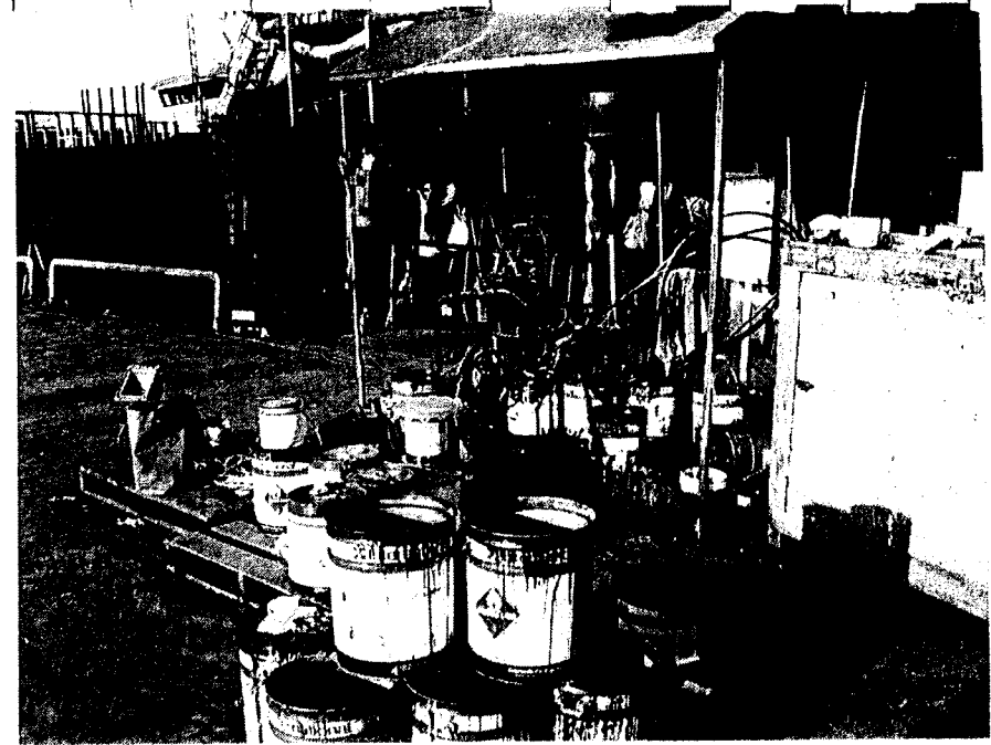
Portable shelter for paint mixing with rain cover and recessed metal floor for containment
