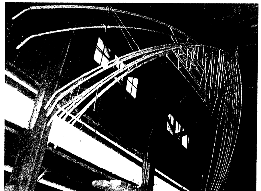
Aluminum arches used to support shrouding of vessel topsides in a drydock
