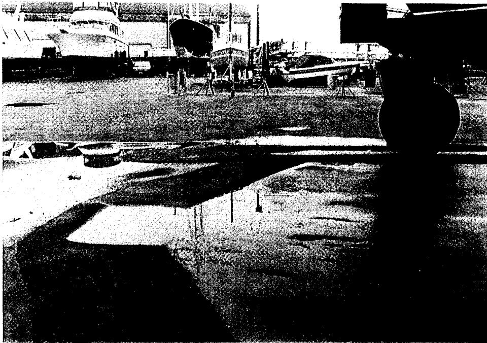
Sloped bermed area to direct hull wash water to sump for sludge catchment
