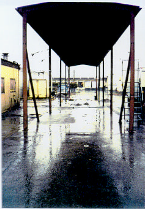
COVERED WASH AREA
