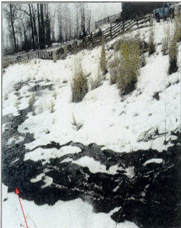
Plate #1: Before Contaminated runoff flows parallel to watercourse. Flow < 30 meters from creek, high impact potential.
