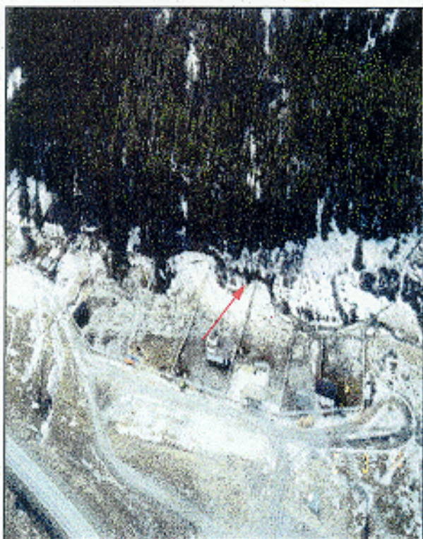
Plate #3: Before Confined livestock areas have access to creek.
