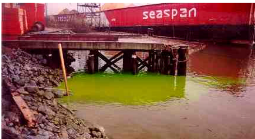
Photo #2: Contaminated Storm water Runoff Discharging into the Fraser River with Fluorescence Dye used to Highlight the zone of Impact.
