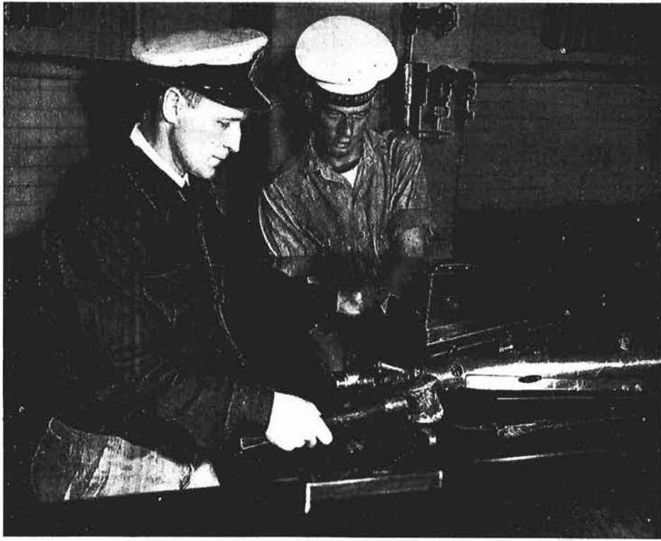
Stripping the tail of a torpedo in the Ordnance Training Centre, HMCS "Stadacona," are CPO E. M. Parker and AB J. F. Connors, both of Halifax, members of the staff of the OTC.
