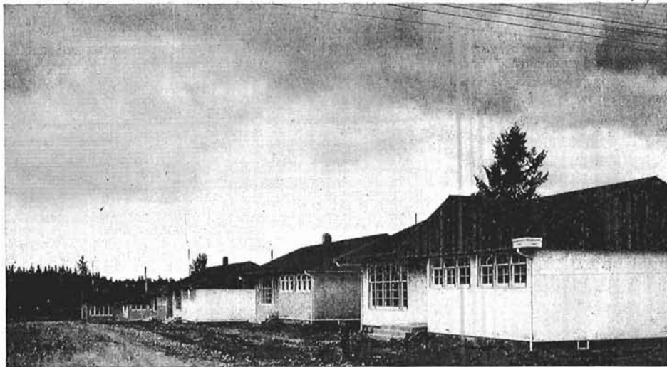
Now near completion are the married quarters at the RCN's radio receiving station at Aldergrove, B.C. This is one of several married quarters projects under way at naval stations on the two coasts.
