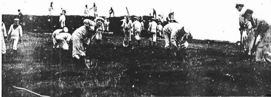
British sailors building the Comox rifle range in 1895. (E-38258)
