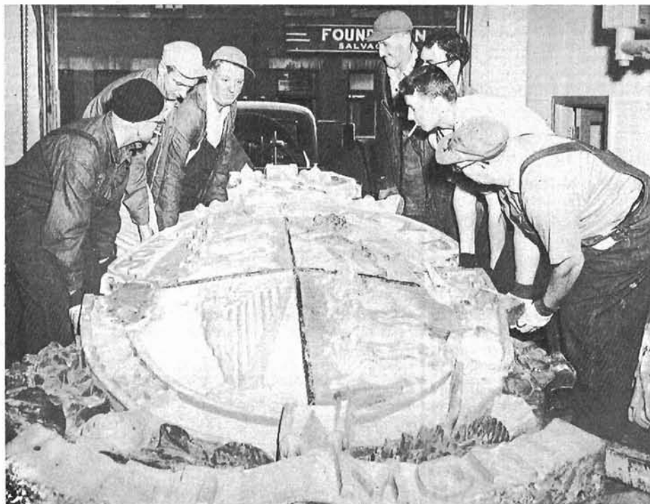
Dockyard employees wrestle the 2,200-pound centre section of the Royal Arms which once adorned the Customs Building onto a flat bed truck to take it from the Ralston Building to the Dockyard for refurbishing and eventual display on a site overlooking the parade square. The Arms, made of bronze, weigh three tons when flanking lion and unicorn are included. (HS-53937)
