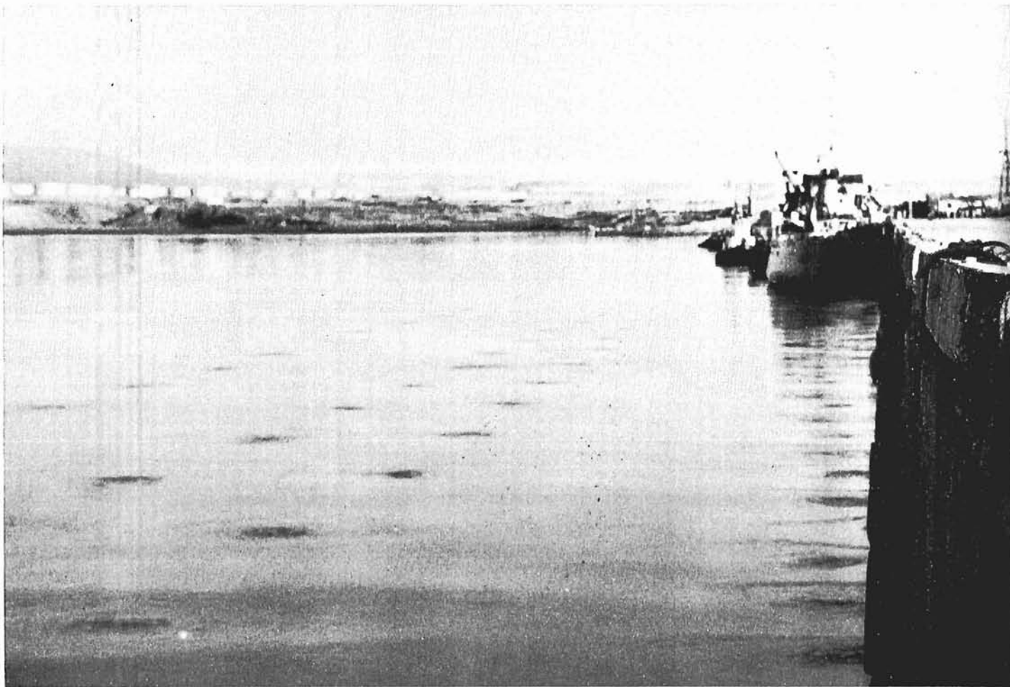
The pattern of disturbed patches on the smooth surface of Thule Harbour, in Greenland, indicates that the polynia system, installed with the assistance of RCN divers, is functioning as it should. The slightly warmer water of the harbour bottom is carried to the surface by air bubbles to prevent the formation of ice. (Official U.S. Navy Photograph)
