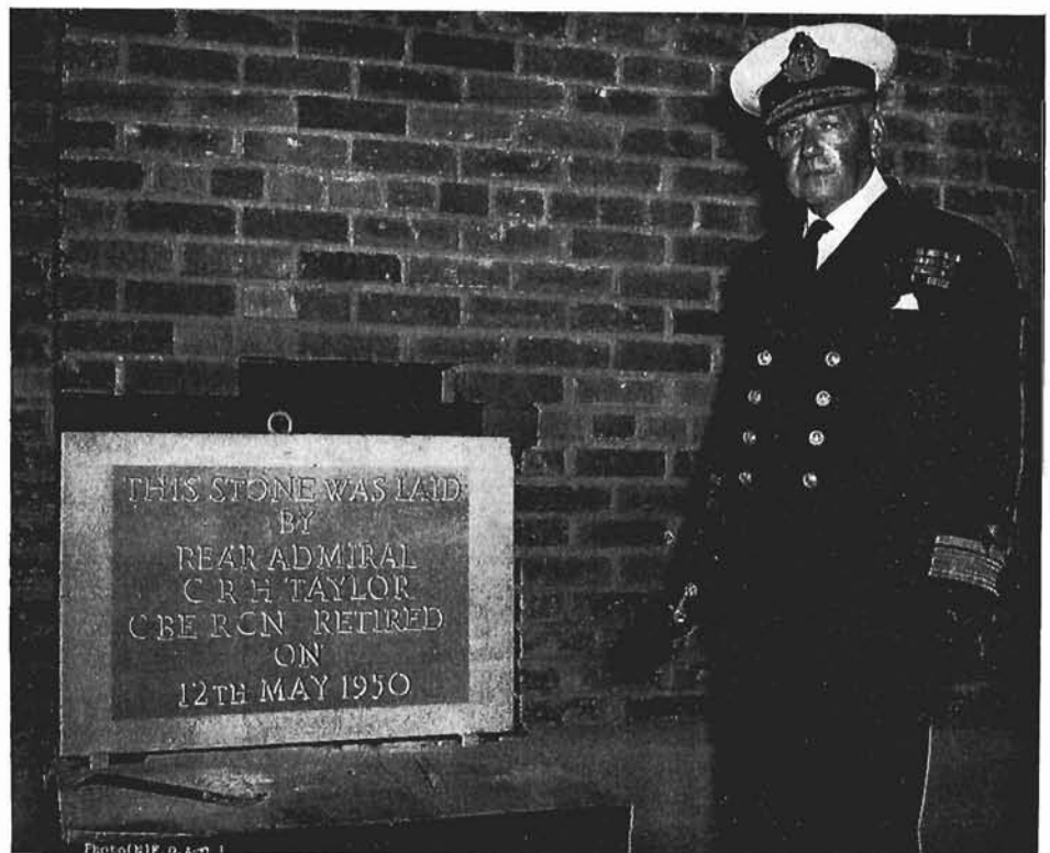
With a tap of his engraved silver trowel, Rear-Admiral C. R. H. Taylor, CBE, RCN, Ret'd., declared the cornerstone of the new "Stadacona" men's accommodation building "well and truly laid." Admiral Taylor campaigned vigorously for the new building during his term of office as Flag Officer Atlantic Coast and it was largely through his efforts that the project was undertaken. (HS-10916.)
