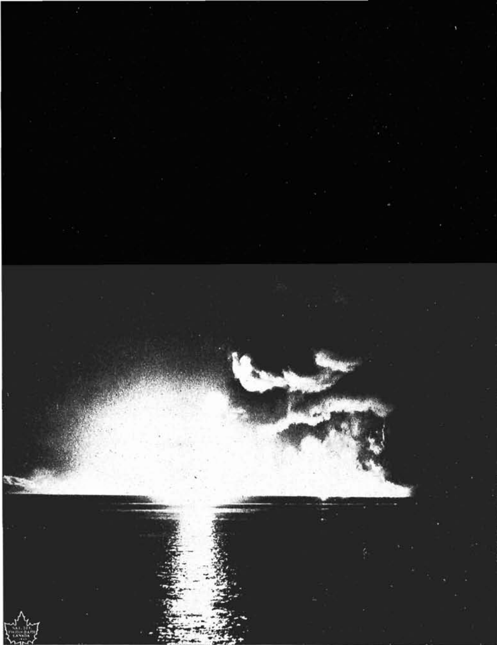
This dramatic photo shows dense columns of smoke rising from oil tanks, supply dumps and other targets blasted by UN destroyers following the Chinnampo withdrawal. (CA-314).
