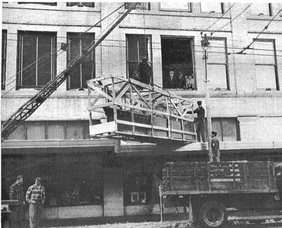
Ever try to navigate a destroyer through a second-storey window? The ship in question was the 40-foot model of HMCS "Iroquois" which went on display on the second floor of Woodward's department store in Edmonton recently. It took a mobile crane and a "berthing party" from HMCS "Nonsuch" to solve the tricky pilotage problem. (Photo by Laddie Ponich, Edmonton).
