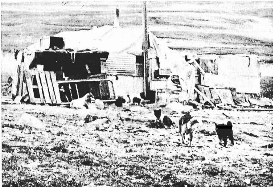
A fine example of modern Eskimo architecture is this Padloping Island bungalow, constructed of canvas, crating, seal skins and even an old bed spring.
