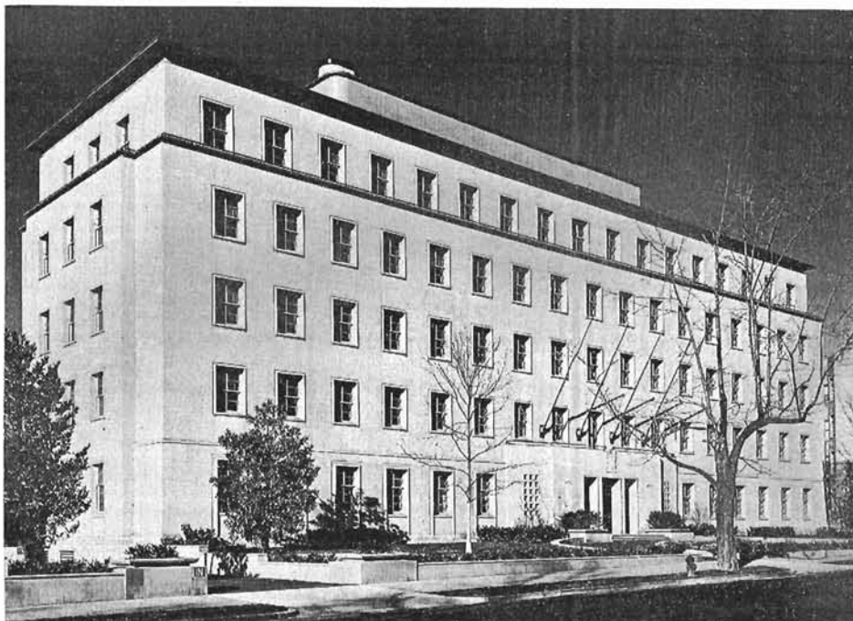
The third floor of this handsome building on Massachusetts Avenue in Washington, D.C., is headquarters for the Naval Member, Canadian Joint Staff, (Washington) and his staff. (Photo courtesy Davis Studio, Washington)
