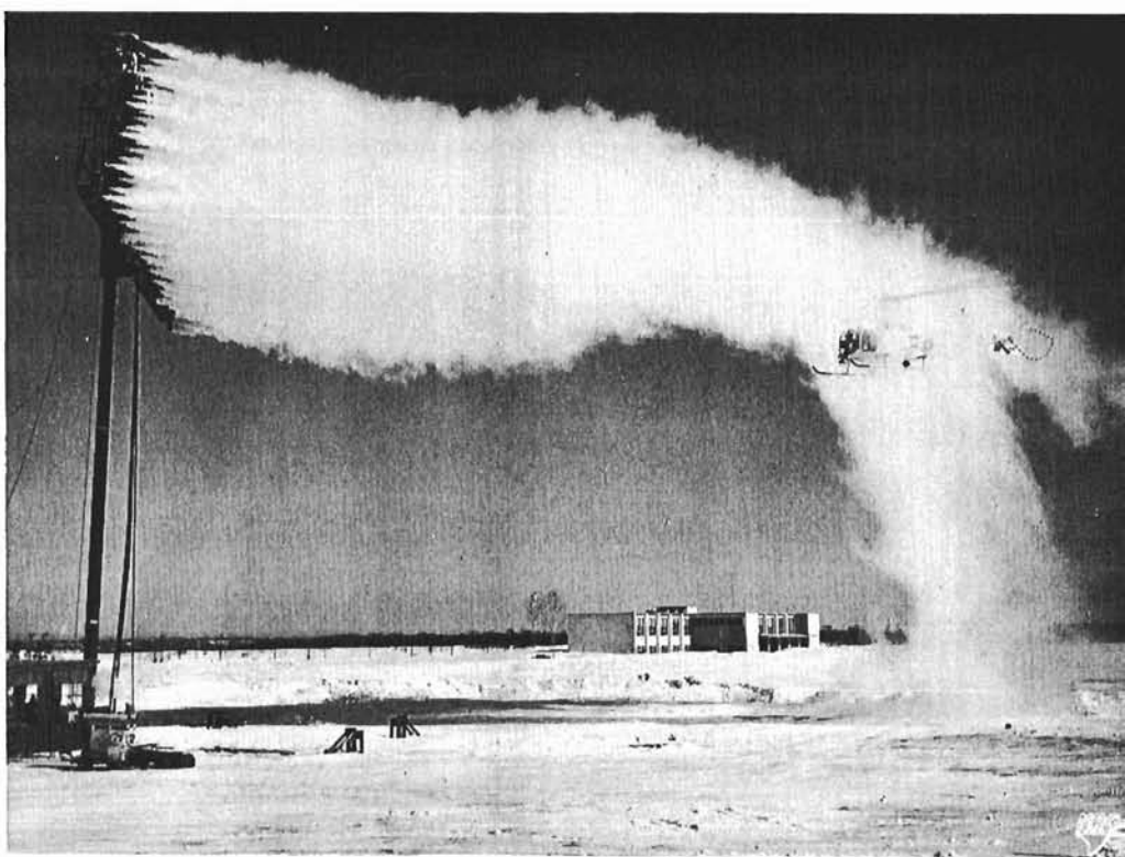
Here is an instance of an airman deliberately trying to get forced down by ice. An RCN helicopter is seen defying the worst that could be done by a freezing cloud produced by an array of 143 fog nozzles during an experiment conducted last winter by the National Research Council in Ottawa. NRC scientists were trying out systems for de-icing the whirlybirds. (Photo courtesy National Research Council)
