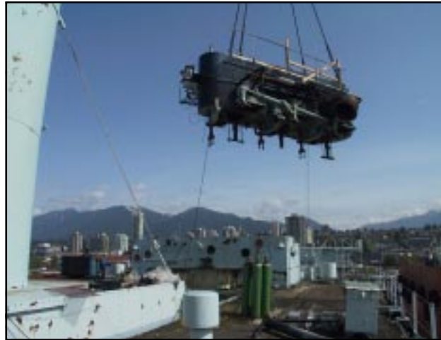
Engine liftout, May 9. HMCS Cape Breton 's three-cylinder, triple-expansion steam engine will become the working centrepiece of a new waterfront museum in North Vancouver. The huge engine weighs 120 tonnes and stands more than two storeys tall. (Photo by Lightstone Video Services)
