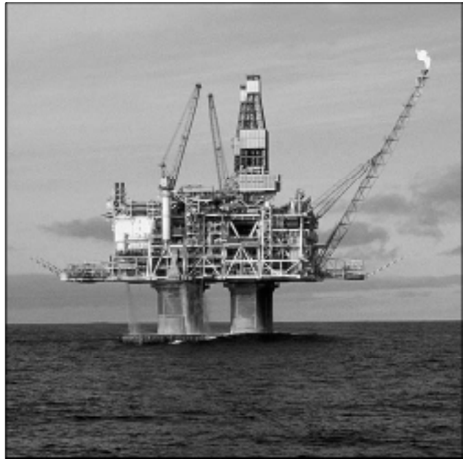
Medium-voltage switchgear has been successfully applied to the power plants of huge offshore platforms such as Hibernia pictured here. (Photo by Hibernia)
