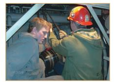
Step 8. FMFCS mechanical apprentice Jake VanRossum (left) and FMFCS rigger Justin Burke rig the new 265-kg clutch in place.
