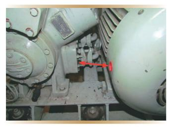
Figure 2. Close-up view of the limited space between the motor and compressor. The oil sight glass is to the left.
