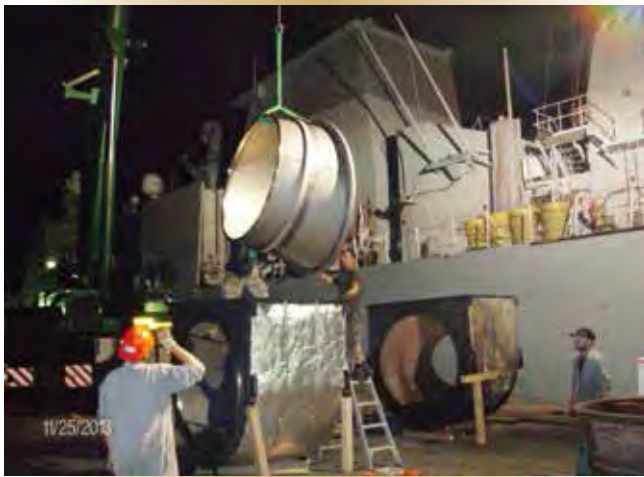
Figure 10 – The work went on 24/7. Here, shoreside, the night shift crew lowers a new diffuser into the new exhaust duct, then installs the unit into the engine enclosure.
