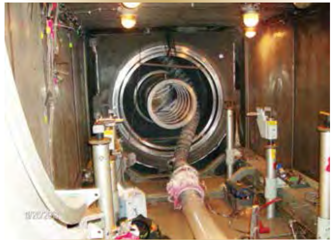
Figure 10 – The work went on 24/7. Here, shoreside, the night shift crew lowers a new diffuser into the new exhaust duct, then installs the unit into the engine enclosure.
