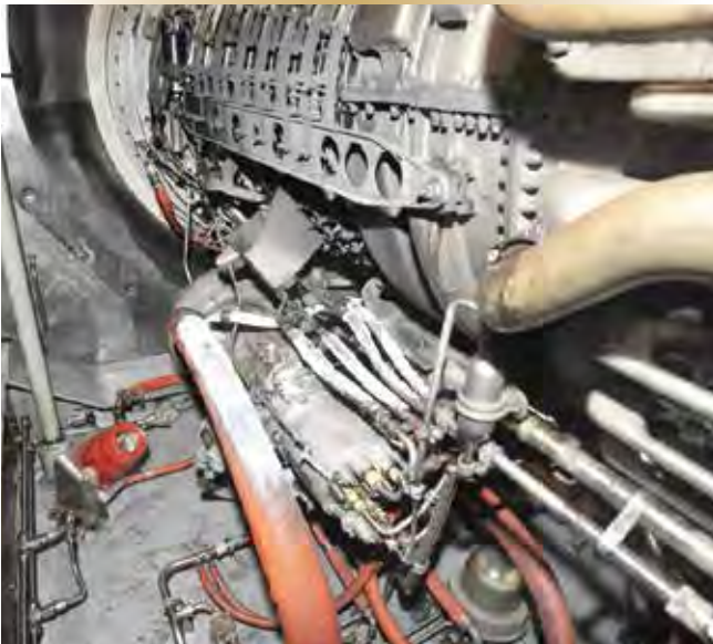
Figure 2 – At first the fire damage appeared to be localized near the fuel pump and main fuel control toward the forward end of the engine enclosure.
