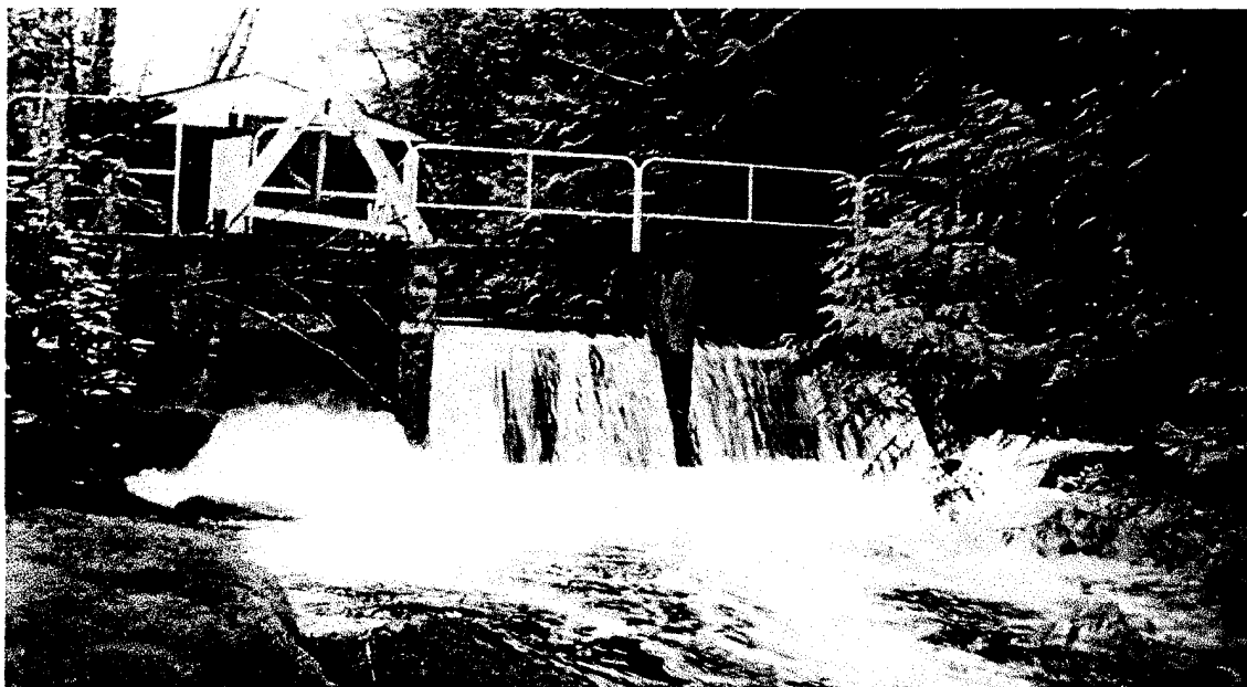
Figure 4. The dam structure located at the outflow of Sakinaw Lake. The structure was constructed around 1957 and has a fishway built into it on the north side.
