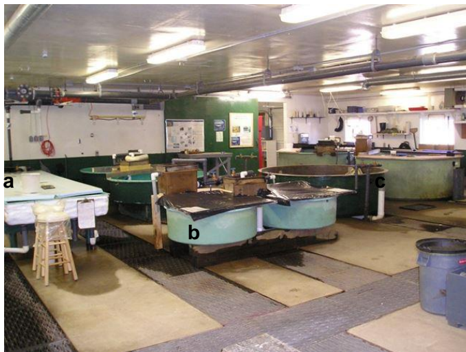
Figure 15. Interior of Mersey Biodiversity Facility, NS. From left to right: a) incubation flow-through tanks, b) larvae rearing tanks, c) broodstock tanks. Illumination from both fluorescent tubes and natural light through windows adjacent to broodstock tanks. Photo courtesy J. Whitelaw, DFO.
