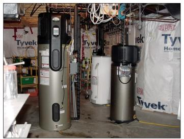
Figure I Heat pump water heaters installed in the basement of the CCHT experimental house. (Left: heat pump water heater A – 80 U.S. gal./303 L, Right: Heat pump water heater B – 50 U.S. gal./189 L)
