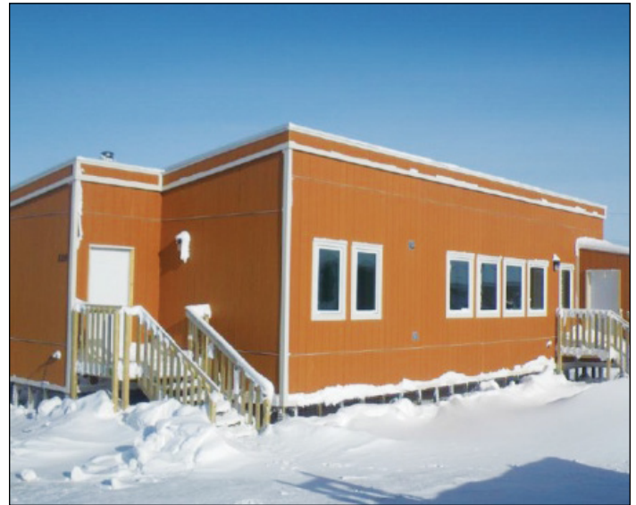
Figure 1 Northern Sustainable House in Arviat (Credit: NHC)
