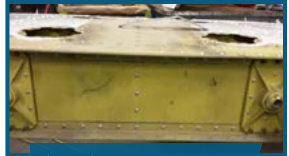
Cracks on the stabilizer rear spar
