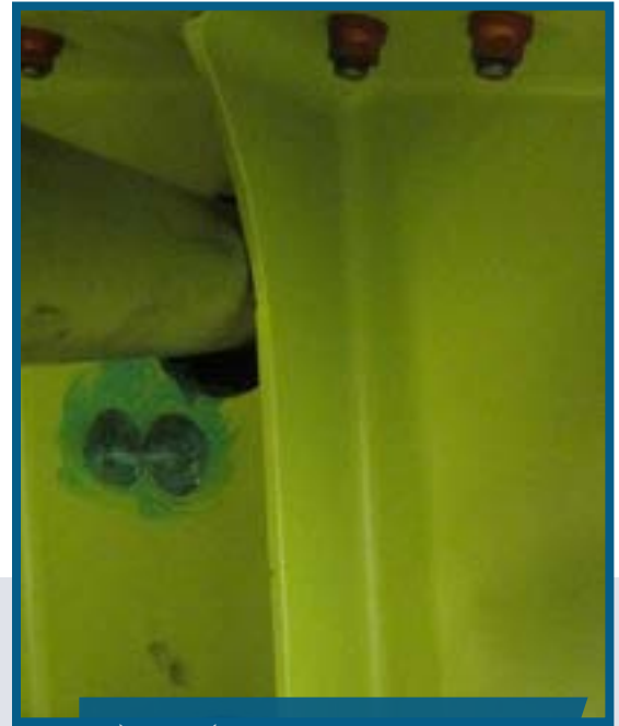
Inner fuel tank line chaffing condition
