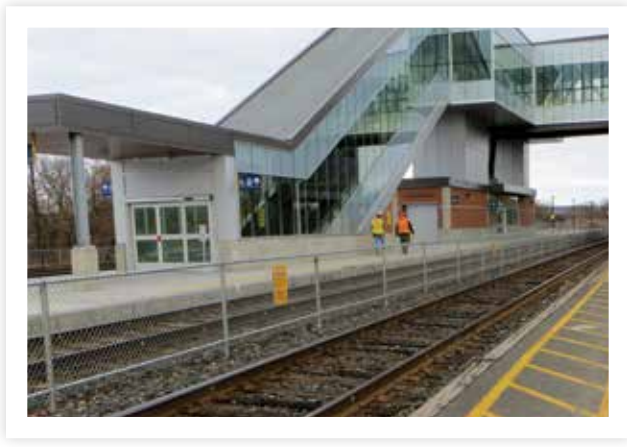
The new overhead walkway at Cobourg Station
