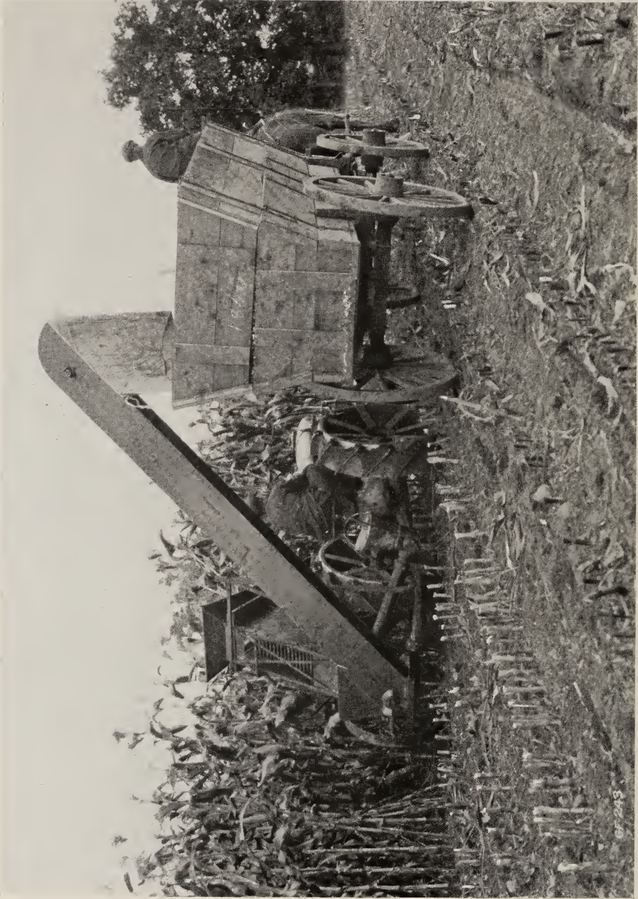
The Roming ensilage harvester. This machine takes the place of the corn binder and silage cutter.
