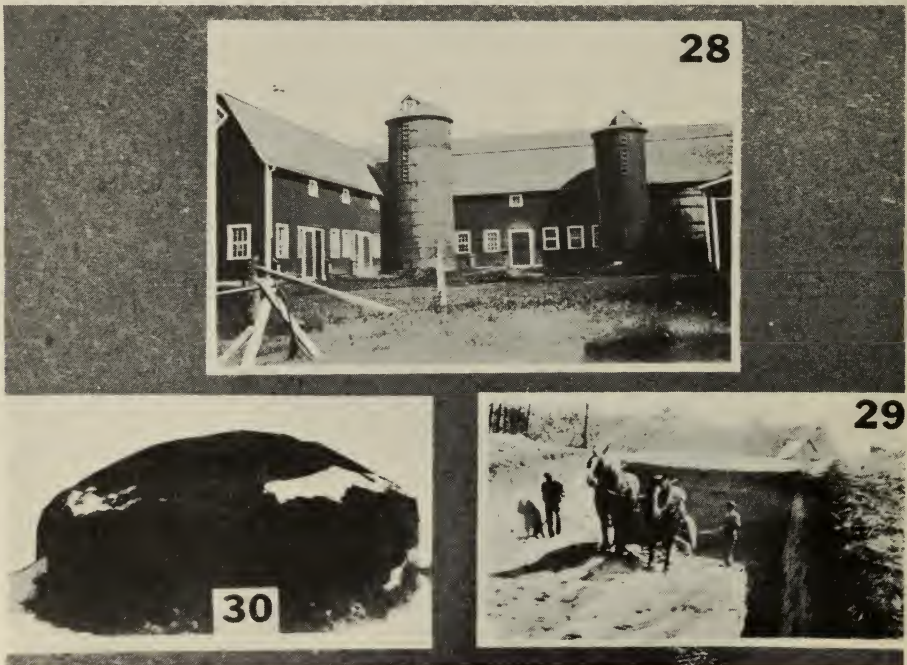
No. 28—Upright type of stave silos in use at the Experimental Station, Lacombe. Silage freezes badly in this type of silo but they are better than other types for spring, summer and fall feeding.
