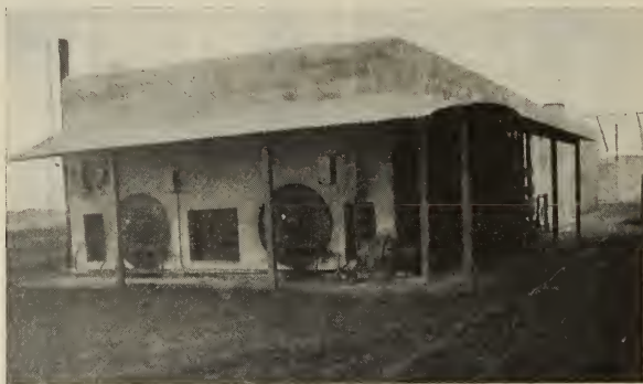
The mechanism of a Miller dehydrator. Note the plastered tile construction, oil burners, and electric motor for fan.
