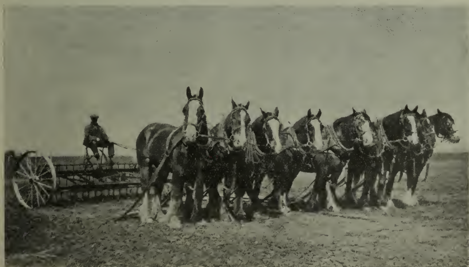
Seed bed preparation or summerfallow can be done at the rate of 25 acres per day with this 11½-foot cultivator.
