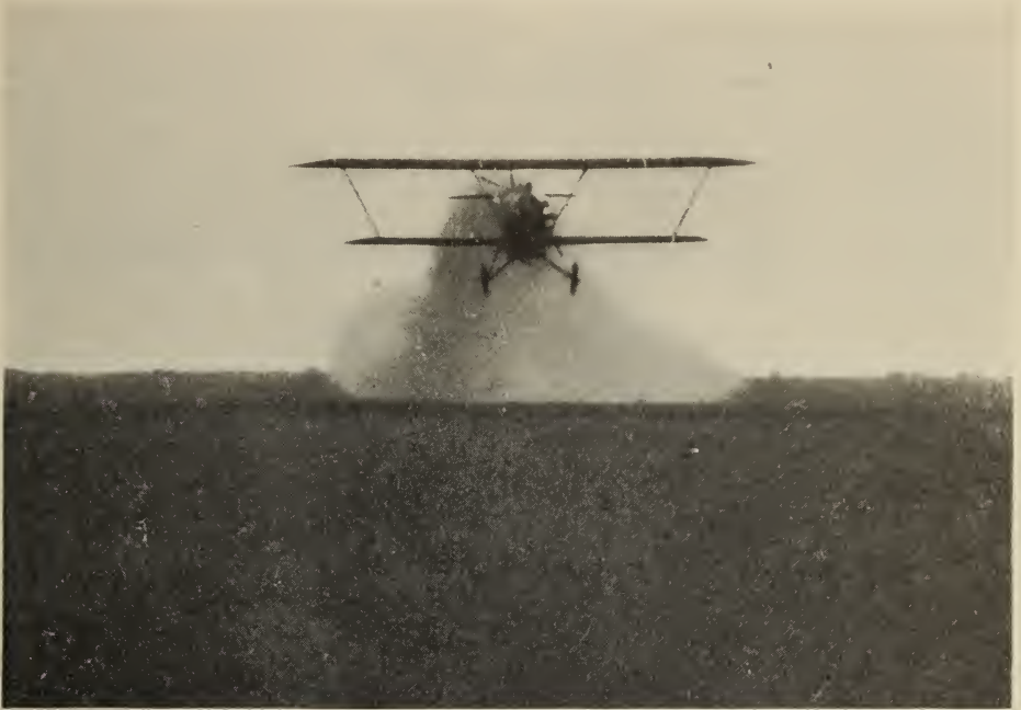
FIG. 29.—Photograph of dusting plane immediately after the hopper-valve was opened. Notice that the dust is forced downward, and due to the rotational flow of air from the propeller it spreads in a spiral arrangement. With favourable air conditions the machine was capable of thoroughly dusting a strip of wheat 100 feet in width.
