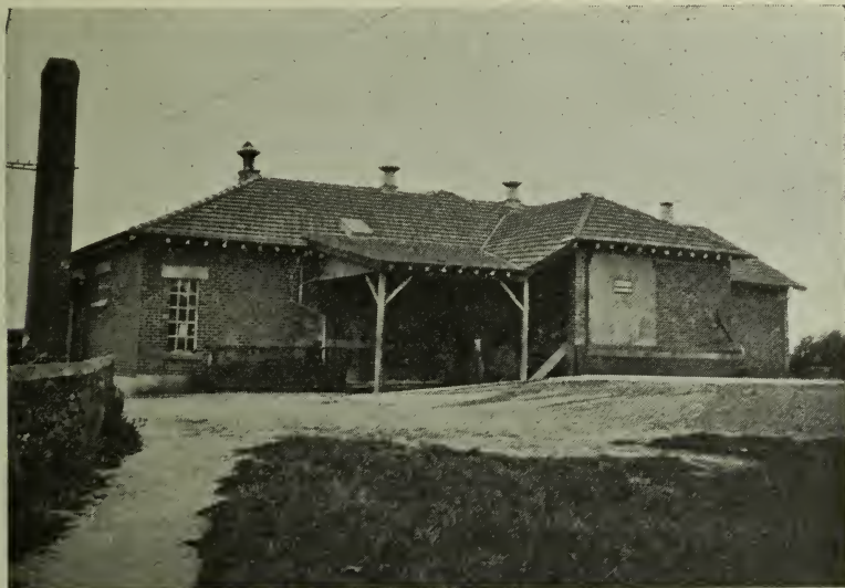
One of the smaller New Zealand cheese factories constructed of brick and concrete with tile roof.
