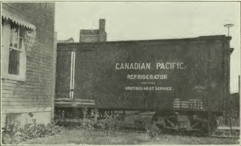
Refrigerator Car. Doors sealed with building paper.
